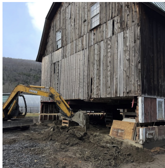
The old 'foundation' being pulled out after the jacking up of the 3,800 sq ft of barn
