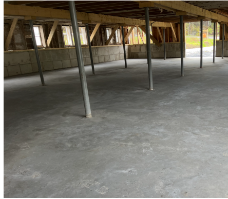
The new floor, interior supports, braces, and foundation wall
